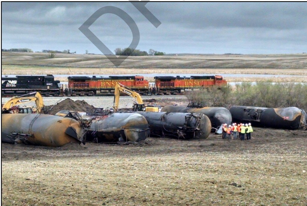
Figure 4.9.2.2 May 6, 2015, Unincorporated Heimdal BNSF Train Derailment
